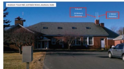
Figure 2. Example of ground-level photograph showing proposed attachment of new equipment.
