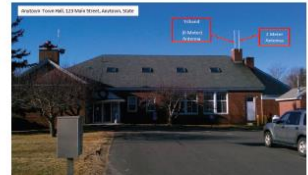
Figure 2. Example of ground-level photograph showing proposed attachment of new equipment.
